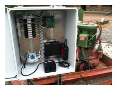
When they began designing the Pump Station Pilot (their next generation lift station product) they selected BTE's Router, Automation Control software, and I/O module to be the basis of their new platform. Using BTE's products, they designed and now manufactures a turn-key lift station product that manages wet well levels by sequencing between 1 and 4 pumps using a wear leveling function provided by BTE's Automation Control. Municipalities using the Pump Station Pilot
